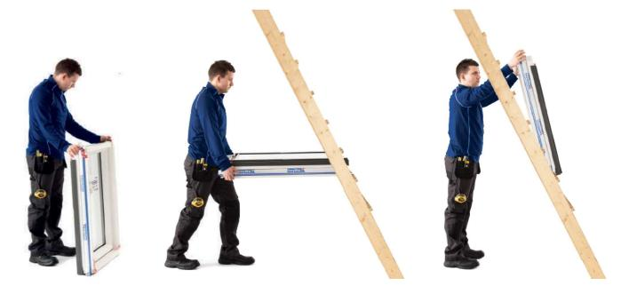
Our Flick-Fit brackets are pre-fitted to our skylights and windows, making them fast and easy to secure into the prepared roof opening.
